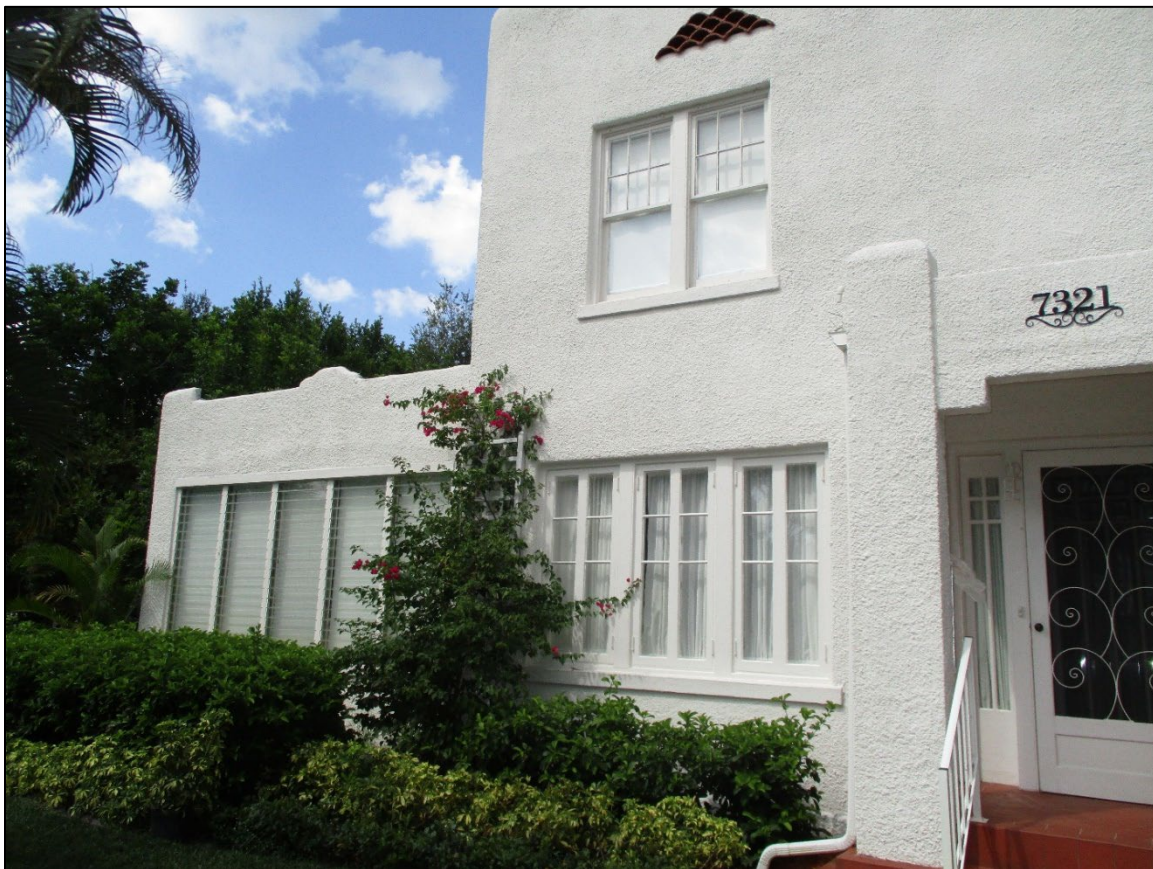
Figure 1: Photograph showing the first-floor French casement windows, second-story six-over-one sash windows, and jalousie windows in the enclosed porch.
